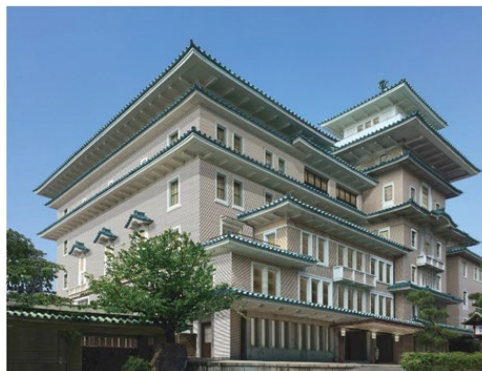
Image: Main Building's southwest exterior
