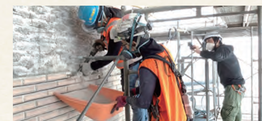
Work to preserve exterior wall tiles at Yasaka Kaikan Hall
